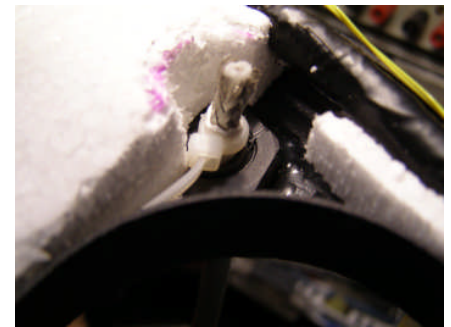
Fig. 9 Coax cable secured with wire tie. Epoxy tail of wire tie to coil housing wall.
